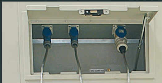
Power Plant Units
